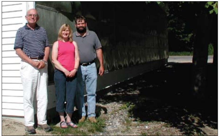
Hancock Energy Advisory Team members (left to right) Selectman John Jordan, Nancy Gamble and Road Agent Kurt Grasset pose alongside the solar panel installed on the town fire station. Photo courtesy the Hancock Energy Advisory Team.
