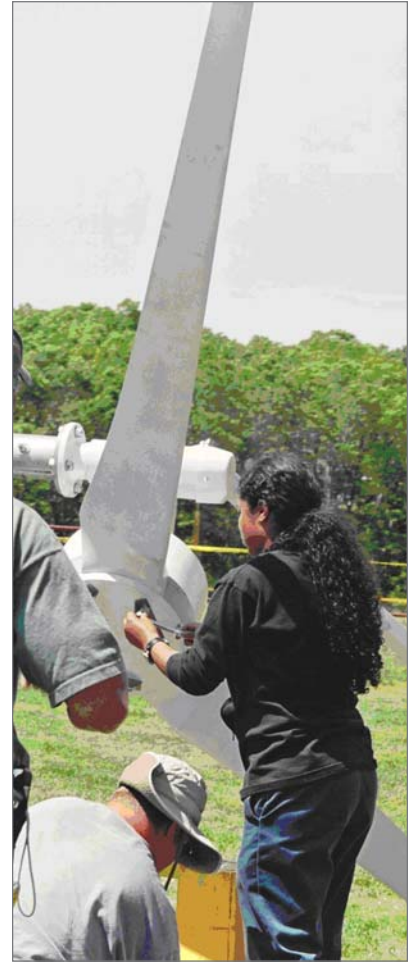
Cape Cod Community College faculty and students install a small turbine.
